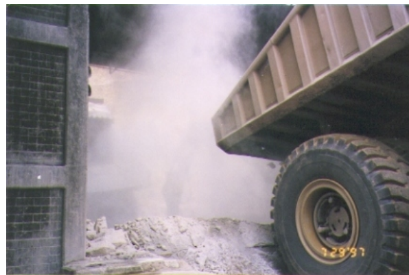
During System Commissioning
